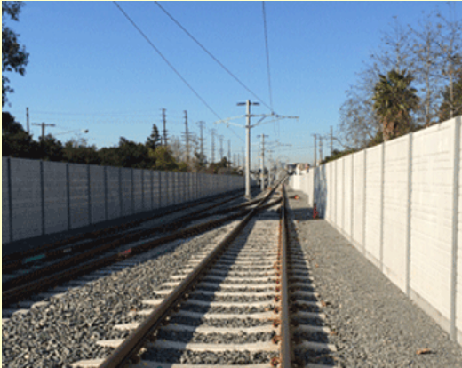
7. This is the right of way between the Westwood and Sepulveda stations. This is the location of the Military Interlocking where there are both facing and trailing crossovers with spring frogs to minimize track noise during normal operations.
