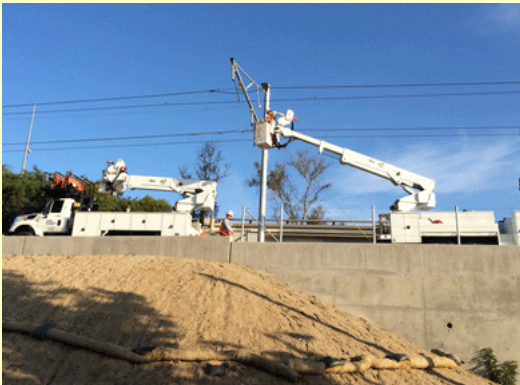
9. During our tour, the crew was working a punch list from a previous MTA inspection. We learned that the catenary is staggered plus or minus nine inches from track center to promote even wear on the pantograph blades.
